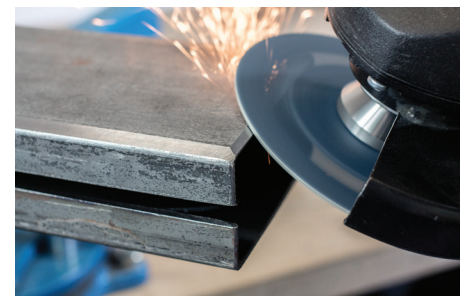
Grind edges ready for welding
