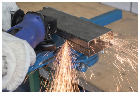
Finishing inside grooves or channels
